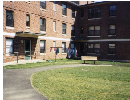
Building Entry & Drying Rack
